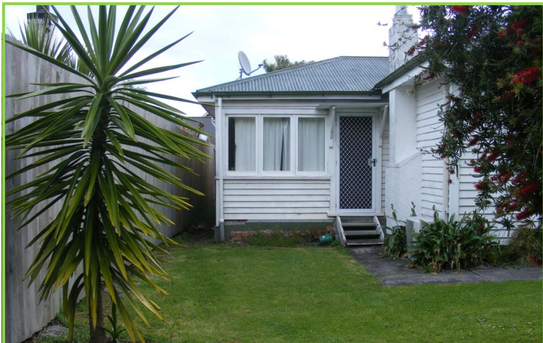
Photo 3: Details of side yard and proposed location of extension.
