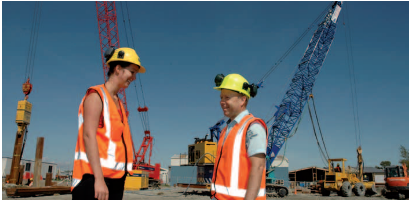
The wastewater treatment plant site at Banks Street is abuzz from dawn to dusk with sheet piling (left of frame) for the three pump stations and the construction of more than 1300 stone columns (right) to support the main structures. Project engineers Sheridan Peckett (HEB Structures, left) and Michael Yukich (Gisborne District Council) discuss progress to date.
