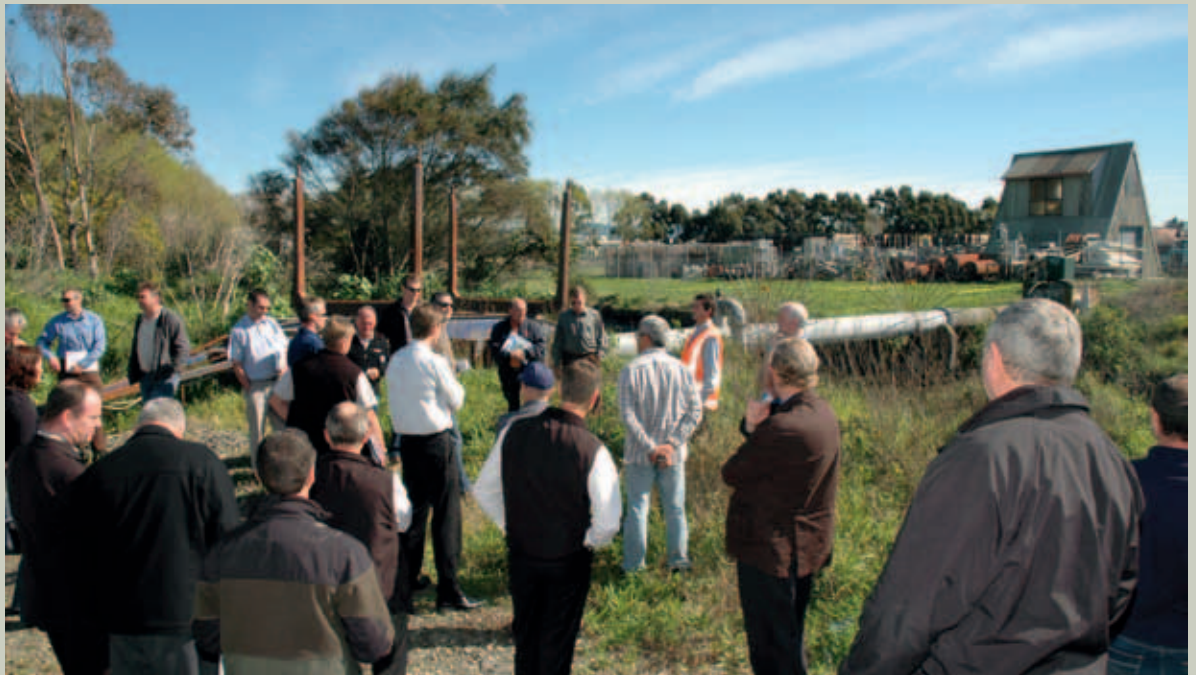
Gisborne Wastewater Project project manager Peter McConnell (hi-viz vest) shows more than 30 contractors' representatives where a wastewater pipe crosses the Waikanae Creek close to the new treatment plant site at Banks Street. The group, representing all companies that earlier registered an interest, were given 36 drawings of the major structures to help them prepare for the tendering process. More than 250 drawings have been prepared by CH2M Beca staff. Part of one building on site has been refurbished to house Council's archives department. A second building will be shifted forward on the site within the next six weeks to make way for construction of the plant.
