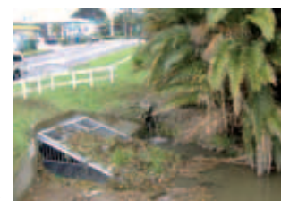
The Hirini Street grille (above) helps trap debris from further up the Kōpuawhākapata Stream (below).
