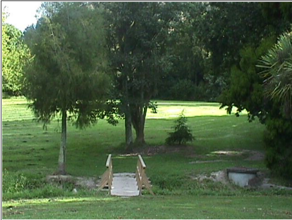
PHOTO 1 : Newly built walk bridge over Waiteata Park Stream. A well known site characteristic of Waiteata Park.
