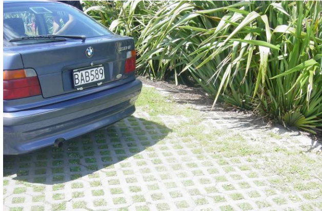
Figure 7: Hard-wearing durable surfaces similar to the above paving option provide necessary protection against earth movement and serve as a softer landscaping feature.
