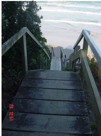
Figure 9: Access A (Tuahine Crescent) stairs.
