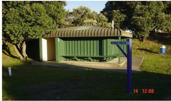
Figure 21: Public Toilets along State Highway 35
