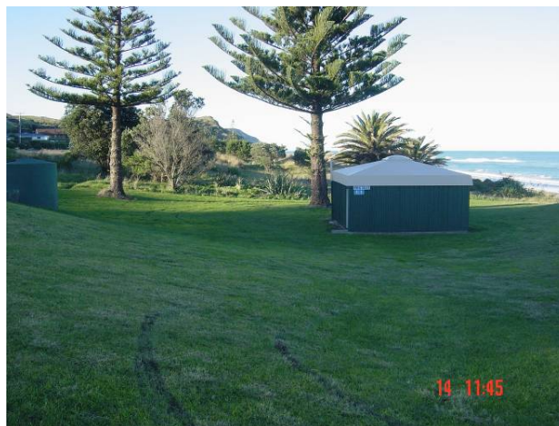
Figure 25: The public toilet from the entrance road.
