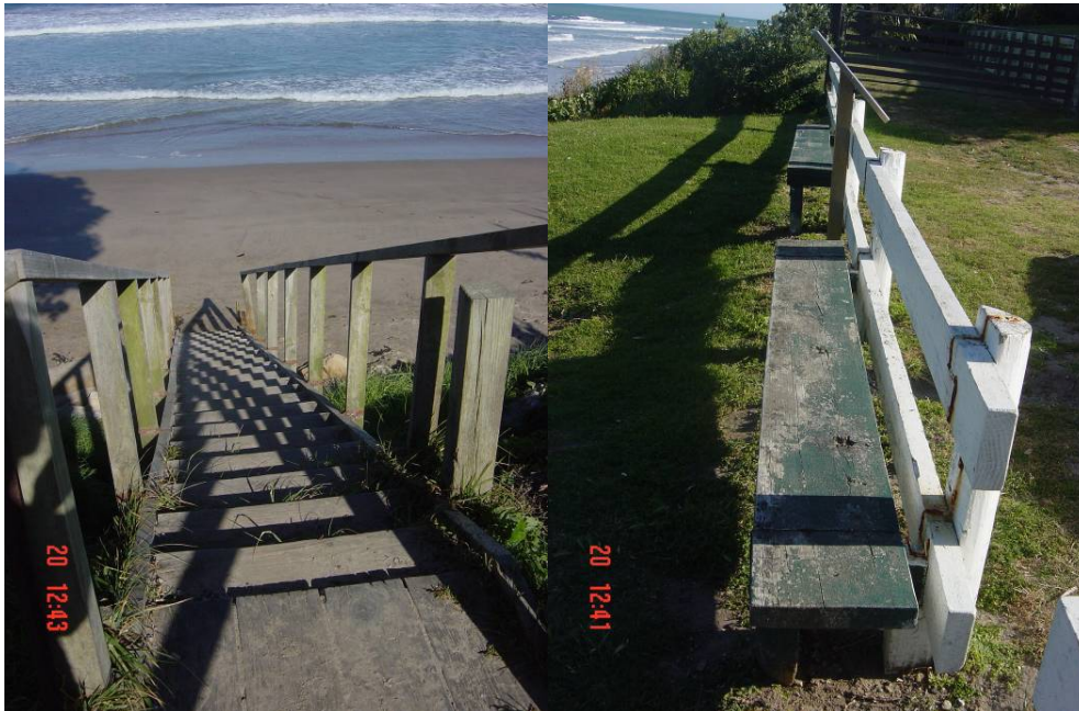
Stairs and fenced access to Wainui Beach from Access B
