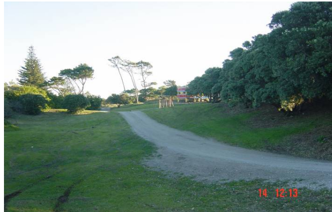
Figure 19: Current metal road joining Access L and M
