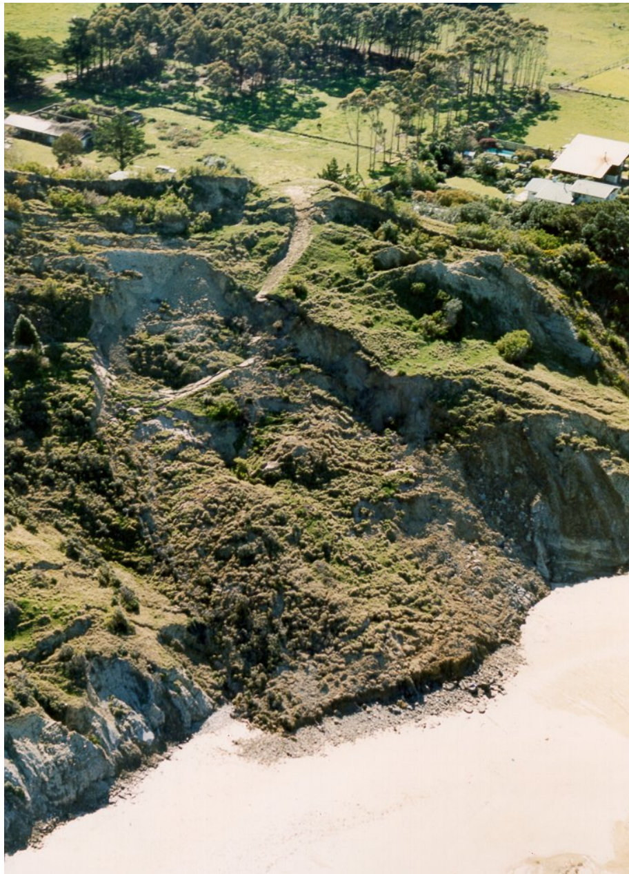
• Figure 14: Oblique aerial photograph taken 19 September 2001 of a landslide near houses at Tuahine Crescent that occurred a few days earlier (Photo courtesy of David Peacock, GDC).
