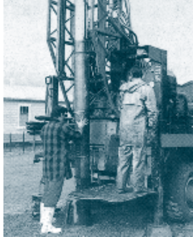
Above: Drilling a groundwater bore is a specialist job.
