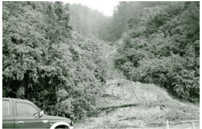
Above: Tauwhareparae Road was blocked by oozing slips for weeks in the spring of 2006.
