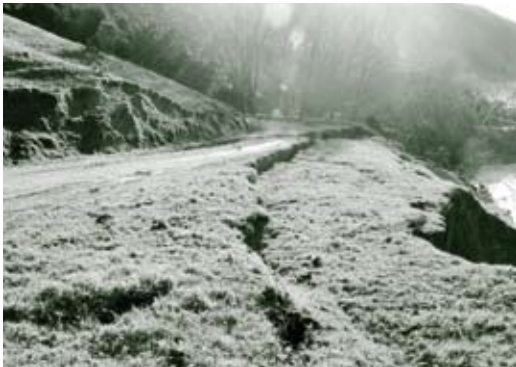
Above: Slumping threatening Shark Bay Road (Anaura Bay). Below: Hore Hore Road completely obliterated by a rock fall. The road was permanently closed.
