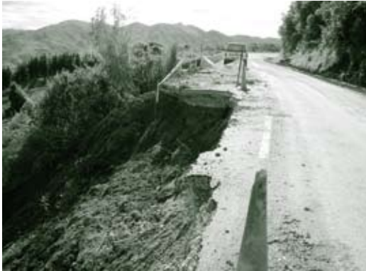
Above: Tauwhareparae Road - severely threatened at Doonholm hill, 2006. Below: Drop out on Mangatu Road.
