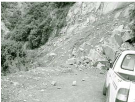
Above: Slumping threatening Shark Bay Road (Anaura Bay). Below: Hore Hore Road completely obliterated by a rock fall. The road was permanently closed.
