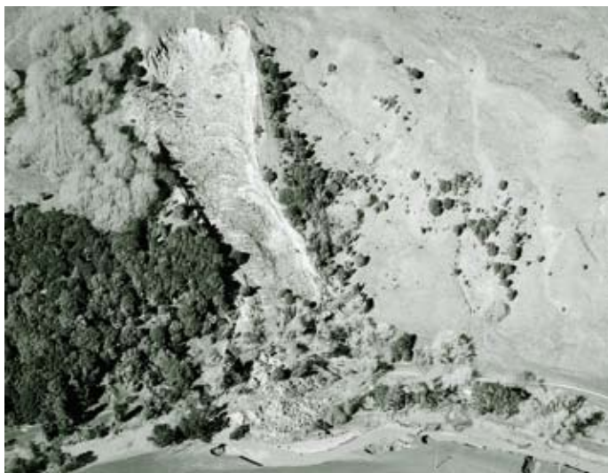
Above: The Waingaromia River flows in its newly-cut channel around the toe of the huge slip, that completely blocked the former channel.
